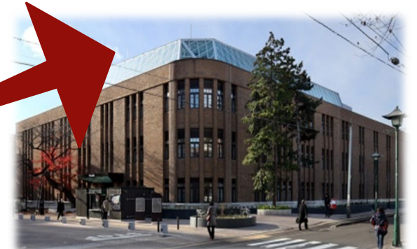
AIMR Main Building
